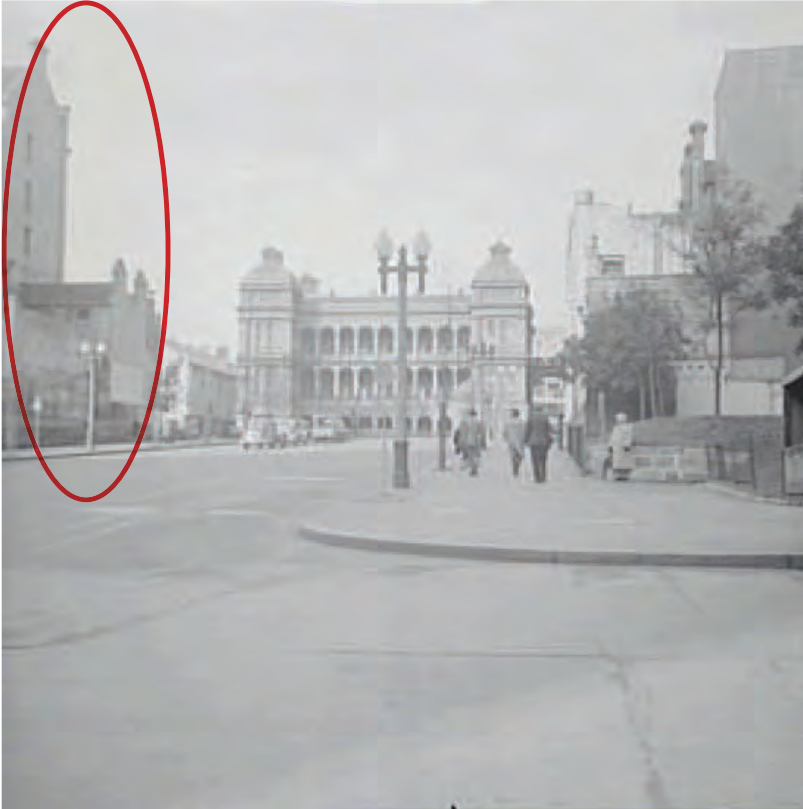
Figure 2.7 Martin Place extended through to Macquarie Street with the Sydney Hospital in the background. The three storey terrace and six storey building to the left of the image are located on the subject site.
