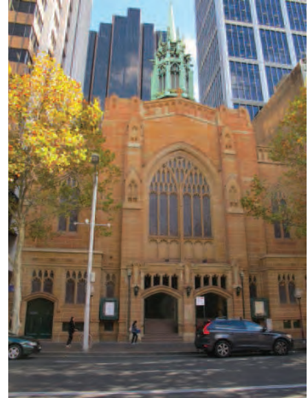
Figure 8.4 Heritage Item, St Stephen's Uniting Church, located at 197 Macquarie Street, Sydney, which adjoins the northern boundary of the subject site on Macquarie Street.
