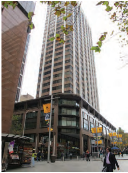
Figure 3.16 The subject site as viewed from west of the intersection of Martin Place and Phillip Street. There is no architectural unity between the tower and the podium of 60 Martin Place. When viewed from this angle the tower appears imbalanced in its relationship with the podium.
