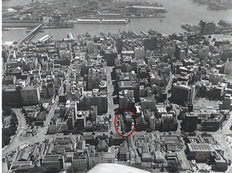
Figure 2.10 An aerial photograph illustrating King Street, Martin Place and Hunter Street. Macquarie Street runs across in the foreground. The subject site is identified with the red circle.
