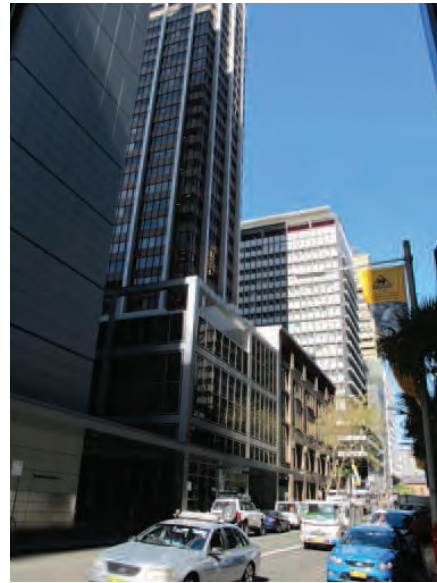
Figure 3.17 The site as viewed looking south along Phillip Street. Significant views to the northern elevation of the RBA building are visible from this angle. There is no architectural unity between the tower and the podium of 60 Martin Place.
