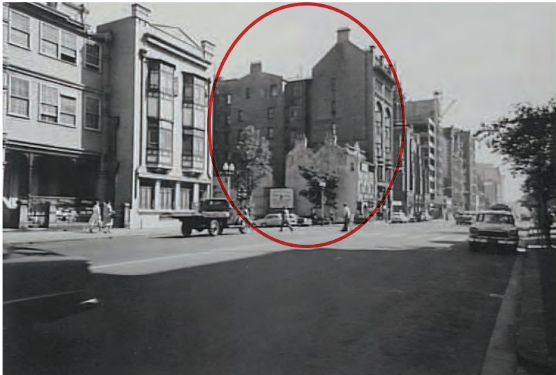
Figure 2.17 View looking north east along Macquarie Street with the Albany (201 Macquarie Street) and St Stephen's Uniting Church to the right of the image. The buildings circled in red in the centre of the image are located on the subject site.
